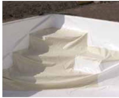
Scala angolo posa liner - Corner stairs laying of the liner
